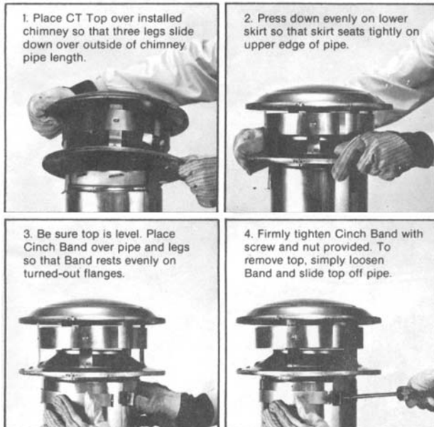
Figure 1 Round Chimney Cap Attachment
